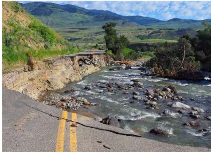
Above: Road Damage in July 2022. Photo by Jenny Golding/A Yellowstone Life.
